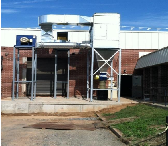
40 HP Drum Storage
