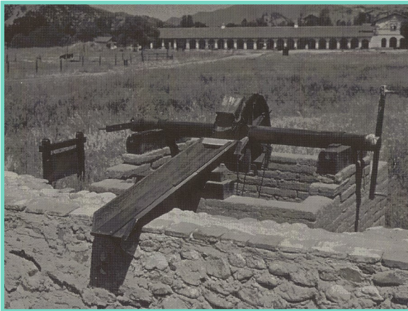
Photograph of the original water wheel at the Noria Well
