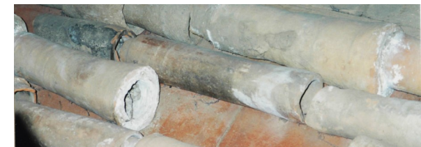
Photograph of the clay pipes used for the water system. They are about 12 inches in length and larger on one end to slip into each other easily. They were laid with great care with layers of tile and rock to prevent pipes from caving in.
