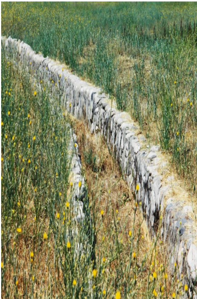
Photograph of the elevated masonry Mill Race
