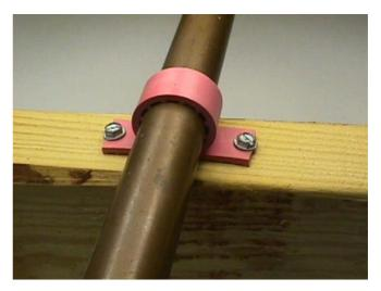
Use on top of joist or rafter and under joist or rafter.
